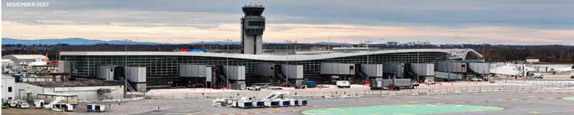
YQB 2018 was highly innovative in its design approach based on Building Information Modeling (BIM)—a first in Québec for a project of its size. The design also reflected a desire to raise the bar for sustainable construction by leveraging geothermal energy, automatic lighting, heat exchange, and fresh air flow control technology.
