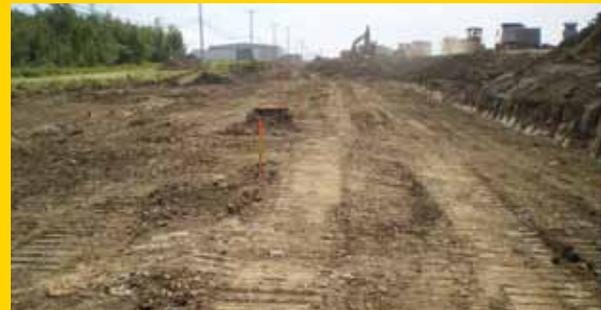
2011 saw the extension of Apron III's paved areas, as well as the gravel surfaces from the Airport's 6<sup>th</sup> Avenue to its 8<sup>th</sup> Street. A lighting system was also installed on the Apron III extension. This work began on June 21, 2011 and was completed on September 23, 2011.
