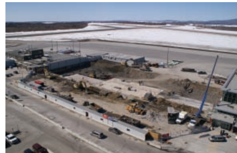
March 28th, 2007, Demolition seen from the control tower
