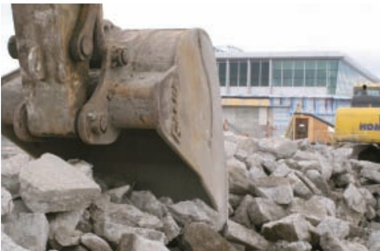
March 23th, 2007, On-going demolition
