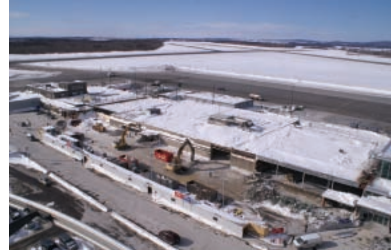
February 23rd, 2007, Demolition seen from the control tower
