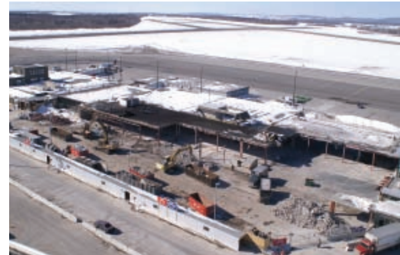
February 27th, 2007, Demolition seen from the control tower
